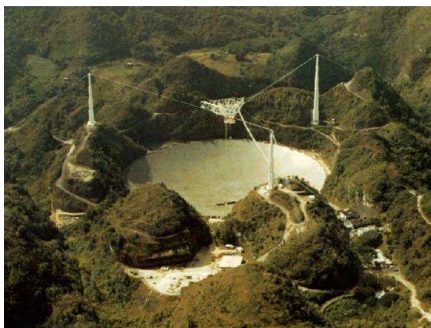
Figure 6.22. Largest Radio and Radar Dish. The Arecibo Observatory, with its 1000-foot radio dish-filling valley in Puerto Rico, is part of the National Astronomy and Ionosphere Center, operated by SRI International, USRA, and UMET under a cooperative agreement with the National Science Foundation. (credit: National Astronomy and Ionosphere Center, Cornell U., NSF)
